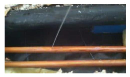
A 1/8 in. leak consumes: 3,806 gal. per day 114,200 gal. per month / At 60psi, a 1/8" hole leaks 296,000 gallons (39,400 cubic feet) in 3 months
