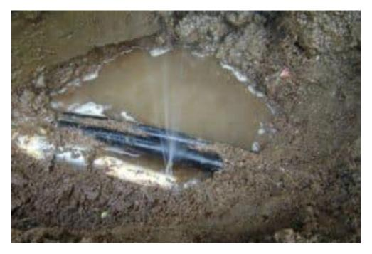
A 1/4 in. leak consumes: 15,226 gal. per day 456,800 gal. per month / At 60 psi, a 1/4" hole leaks 1,181,500 gallons (158,000cf) in 3 months
