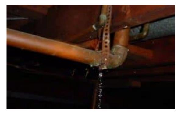
A 1/16 in. leak consumes: 943 gal. per day 28,300 gal. per month / At 60psi, a 1/16" hole leaks 74,000 gallons (9,850 cubic feet) in 3 months
